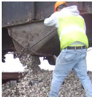
Unloading ballast at Jeff Yard
