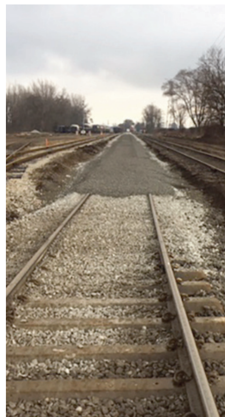
Construction of a new 2,000-foot second-track was completed in December.
