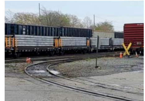
The wye at Fresh Pond
