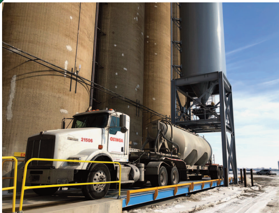
Major improvements and new facilities have been added by Omni at its IIPD terminal, including this weigh scale and loading tank. A new scale house was also constructed, including significant technology upgrades.
