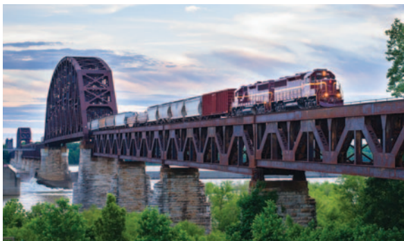
LIRC on the Ohio River Bridge
