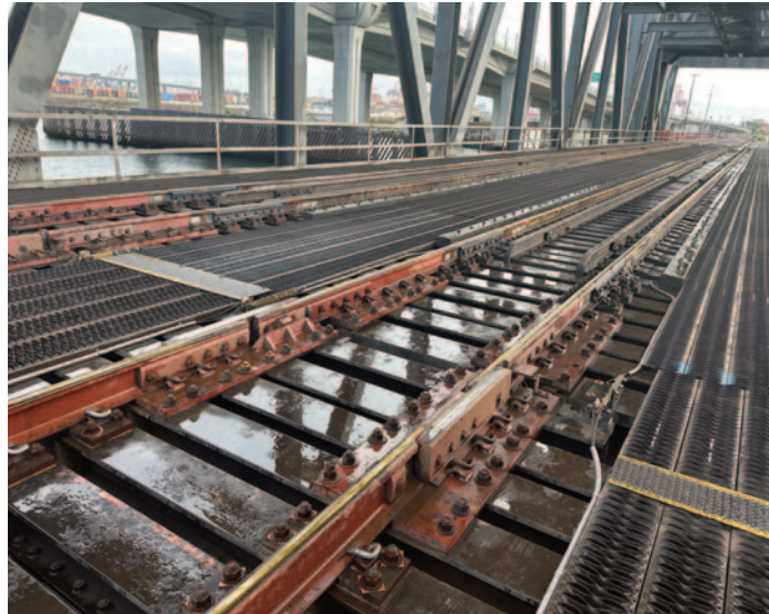
Above: New 136-lb continuous welded rail replaced jointed rail on both tracks.
