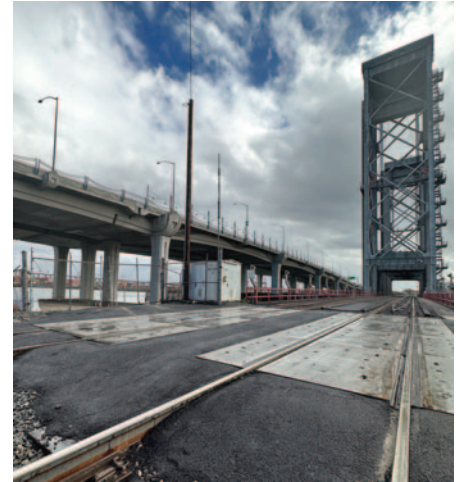
Above: New 136-lb continuous welded rail replaced jointed rail on both tracks.
