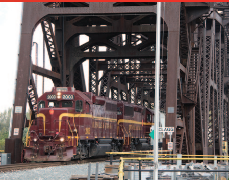
Upgrades continue in 2023 to the Ohio River bridge.
