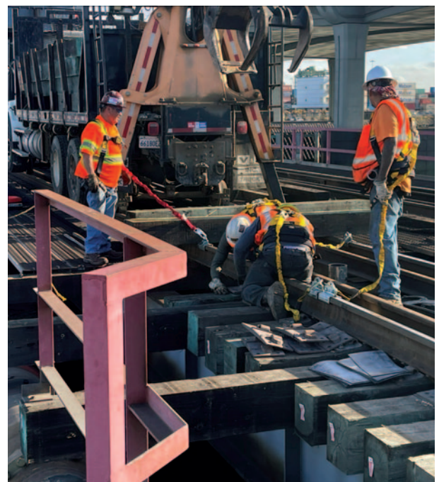
Badger Bridge renewal continues
