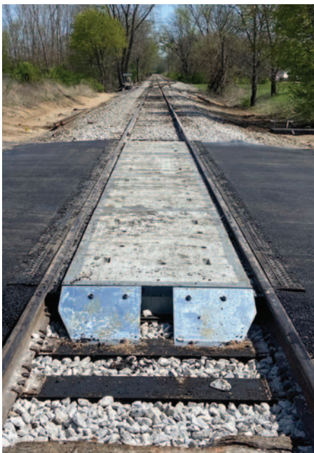
One of the 19 crossings that have been replaced on LIRC this year.
