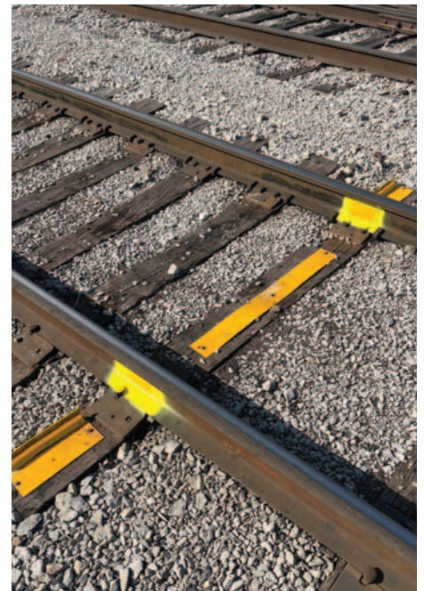
Reflectorized clearance tabs are now in place at every key clearance point in our main Jeffersonville yard.
