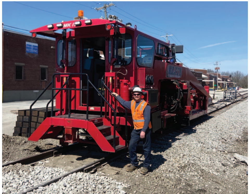
Modern automated track surfacing equipment is used on LIRC, making the work safer, faster, and better.
