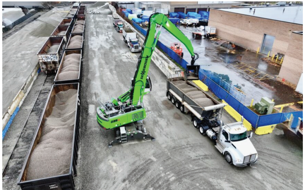
Crushed stone is offloaded from rail cars at Astro Aggregates Hicksville facility. / Courtesy of Astro Aggregates
